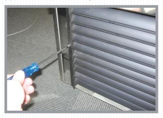
(c) Turn knob on dial to new setting. Never set higher than 75°C. Only adjust dial that is not siliconed. DO NOT remove or adjust siliconed dial.
