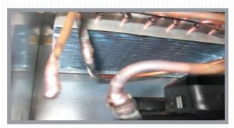
This shows a small condenser which can be accessed from side panel. ENSURE ALL power off and DISCONNECTED and give a clean once every while depending on ambient conditions i.e., dust, open-front door of shop/canteen etc.
